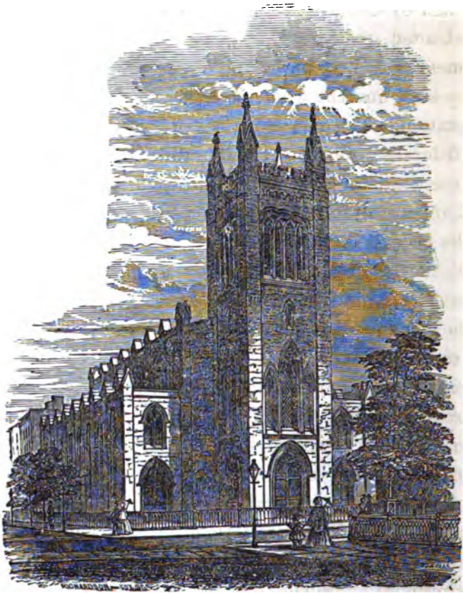
Church of the Ascension, corner of Fifth Avenue and Tenth Street.
